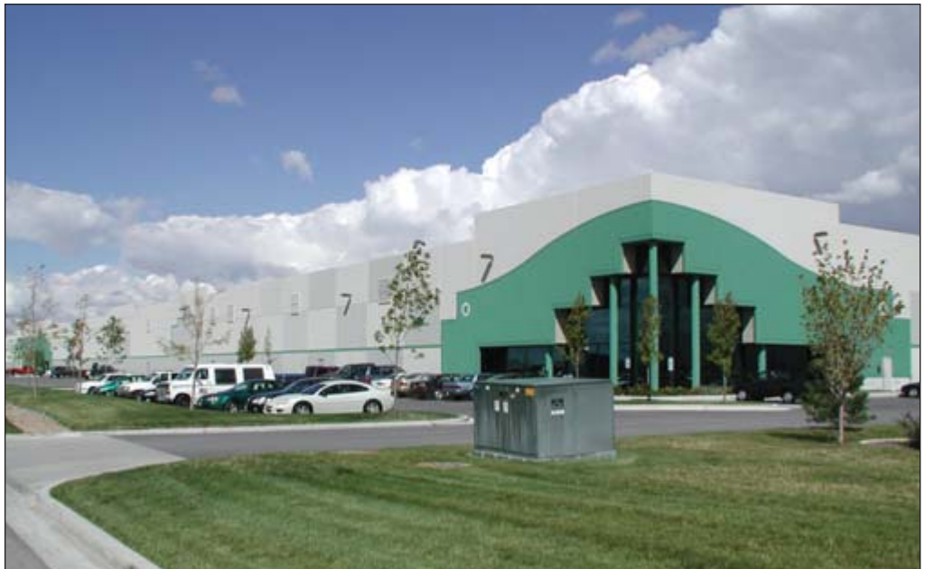
A warehouse in Ninigret Park in Salt Lake City.
